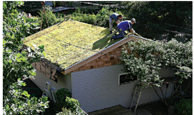
Garage green roof, MarcyHolmes Neighborhood, Minneapolis
